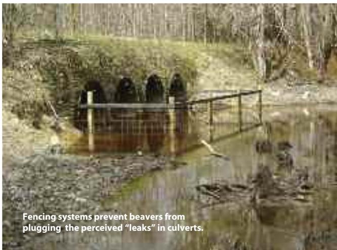
Fencing systems prevent beavers from plugging the perceived "leaks" in culverts.
